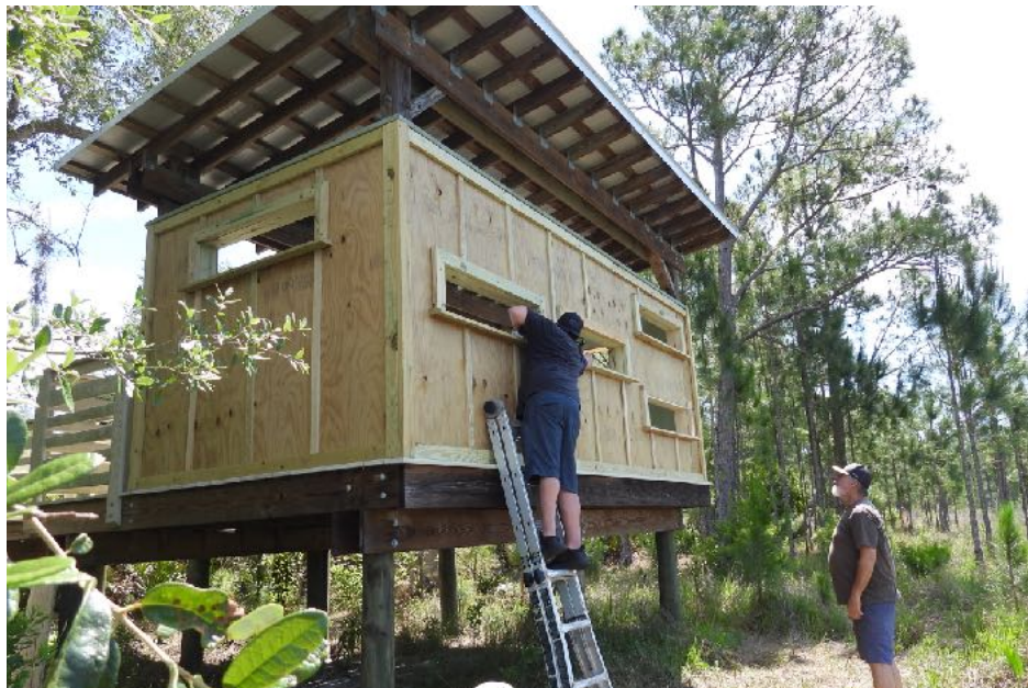
Exterior Work in Progress
